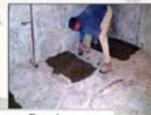
Figure 4 Immediate work area is filled in with new concrete
